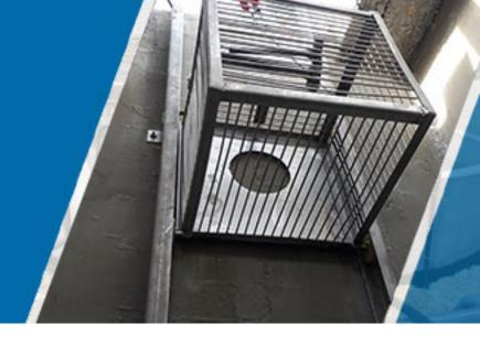
Basket screens are quite simple and low-cost equipment, often used in small-scale treatment plants. Basket screens are used as pre-treatment to protect the equipment behind the line against possible damage and increase the efficiency of the treatment pro-
